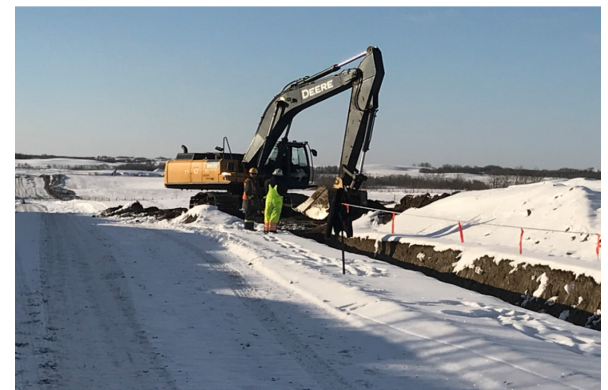
11. Tie in Backfill – Km 28+900 – Nov 8, 2017
