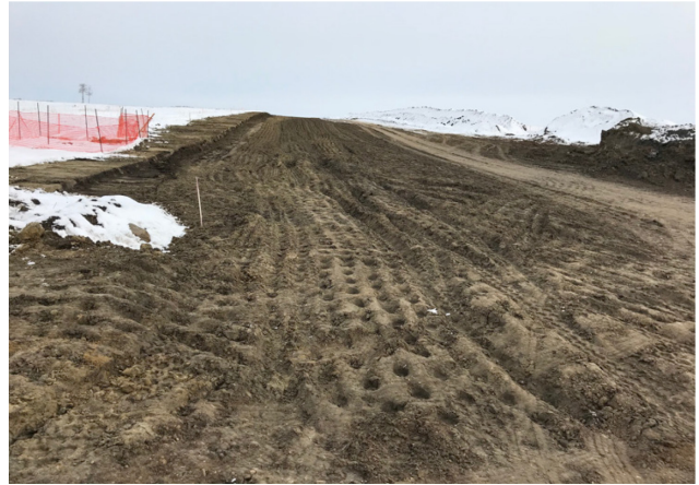
8. Tie in work complete – Km 43+600 – Nov 7, 2017
