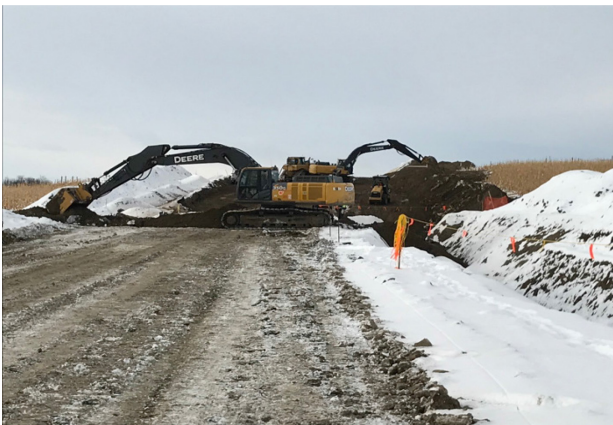
5. Tie-in Backfill – Km 30+750 – Nov 7, 2017
