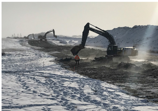
9. Tie-in Backfill – km 58+900 – Nov 8, 2017
