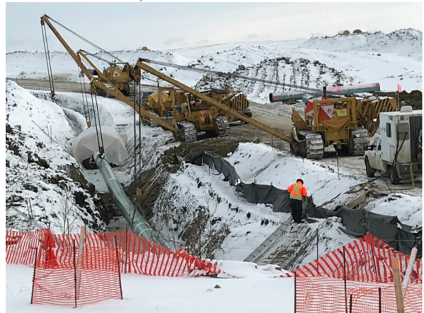
4. Tie in work – Km 33+900 – Nov 7, 2017
