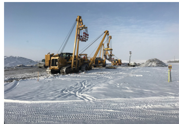
10. Lowering Crew – Km 59+900 – Nov 8, 2017
