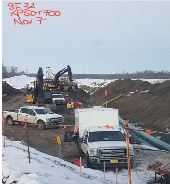
14. Excavating – Km 50+700 – Nov 7, 2017
