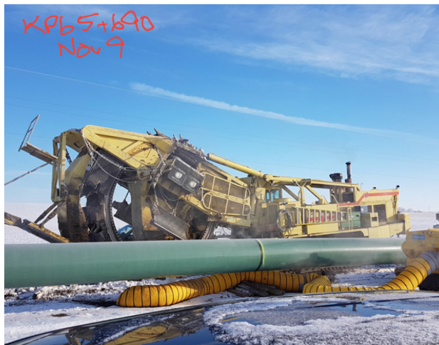
15. Ditcher Maintenance – Km 65+690 – Nov 9, 2017
