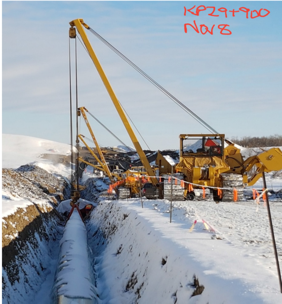
13. Backfill – km 29+900 - Nov 8, 2017
