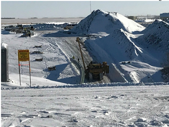
3. Bending Crew – Km114+400 –Nov 6, 2017
