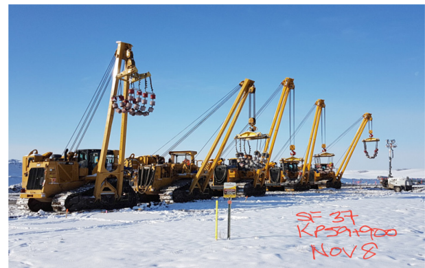
12. Lowering Crew – Km 59+900 – Nov 8, 2017
