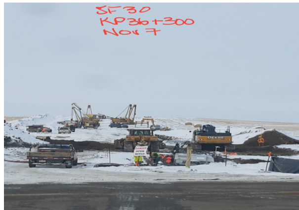
6. Tie in activity – km 36+300(SF 30) – Nov 7, 2017
